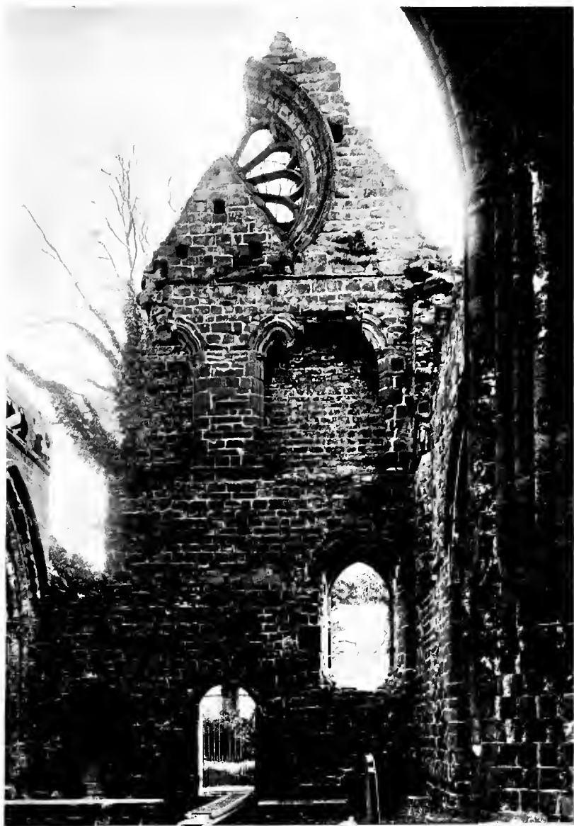
FIG. 150.—South Transept, New Abbey : Interior (No. 380).
